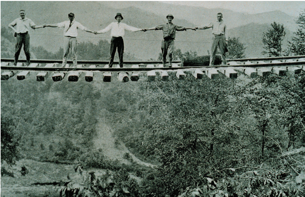
Fill material slid down the mountain, leaving track suspended during heavy rains.
