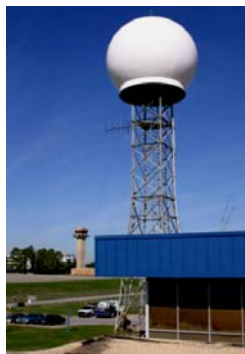
Figure 1. ARMOR radar at Huntsville International Airport.
